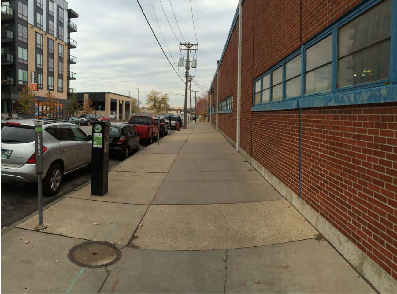
Figure 3.13 Local Commerce Corridor, existing conditions, photograph by the City of Minneapolis
